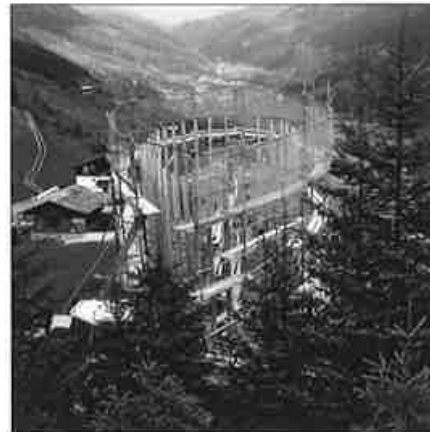
The assembly of the timber structure
